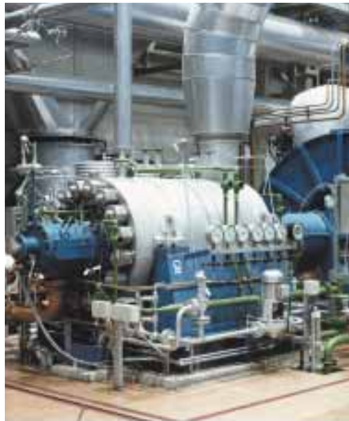
► Boiler feed pump (KSB, CHTA) with a Burgmann type SHV1/200-E1 mechanical seal. ( p_1 = \dots 30 bar; t_1 = 190 °C; n = 5,020 min -1 ; v_g = 57 m/s)
