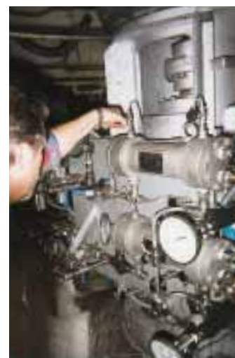
Boiler circulation pump (Halberg) in the Paka combined power station (Pasir Gudang, Malaysia) sealed with type SHPV2/90. ( p_1 = 75 bar; t_1 = 288 °C; n = 1,450 min -1 ).
