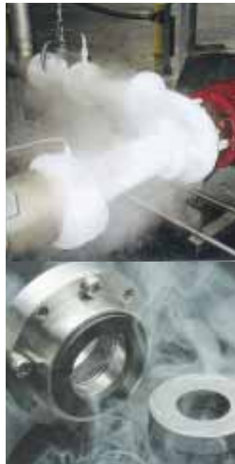
Nitrogen pump in a loading station run by Linde AG. The gas-lubricated MFLC-GS seal from Burgmann has been running without trouble since April 1998. p_1 = 5 bar; t = -196 °C; n = 2,950 min -1 . Further mobile pumps ( n = up to 11,000 min -1 ) in tanker trucks are also being successfully sealed with the MFLC-GS.
