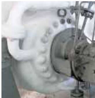
Return pump with tandem seal type H75S2-H75F1 according to API 682 Plan 52 for the sealing of hydrocarbon. Buffer medium: methanol. Temperature: -13 °C.
