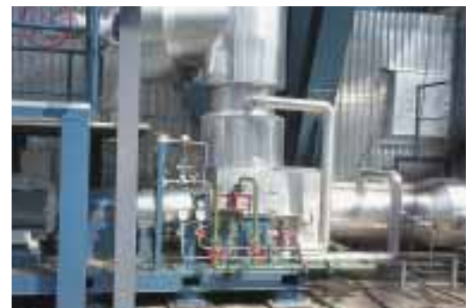
Boiler circulation pump (Halberg) in the Paka combined power station (Pasir Gudang, Malaysia) sealed with type SHPV2/90. ( p_1 = 75 bar; t_1 = 288 °C; n = 1,450 min -1 ).
