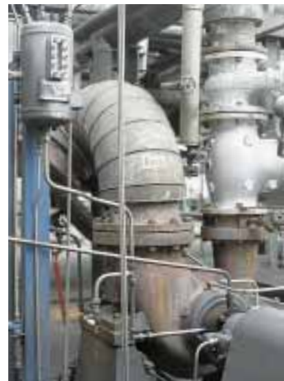
Burgmann mechanical seal type MFLW85S20 for sealing gas oil with sulfur in a Ruhrpumpen pump. Temperature 217 °C, pressure 2.3 bar.
