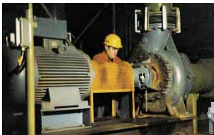
Non-clogging pumps (KSB, KWP) with Burgmann type MFL85N mechanical seals ( Q_{12}Q_1, V T_6G_1 ) in a 5-stage biological sewage works run by DEA Union-Kraftstoff AG, Wesseling, for the biochemical elimination of nitrogen in ammonium-enriched refinery waste water. The useful life of these seals in dead-end arrangement is between 3 and 4 years in the 30 pumps installed at the works. ( d_1 = 53 \dots 90 \text{ mm} ; p_1 = 2 \dots 4.5 \text{ bar} ; t = 20 \dots 40 \text{ °C} ; n = 950 \dots 1,450 \text{ min}^{-1} ).
