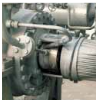
Pump (Ruhrpumpen) with Burgmann tandem seal type H75S2-H75F2 according to API 682 Plan 52. Medium: C 3 fraction; buffer medium: methanol.
