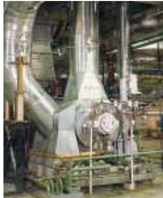
Main feed pump (CCM Sulzer) at St. Laurent nuclear power station (EDF, France). Equipped with a Burgmann type HSHFB 11/191 seal and WE 120 heat exchanger. ( p_1 = 28 bar; t_1 = 188 °C; n = 4,610 min -1 ; v_g = 48.2 m/s)
