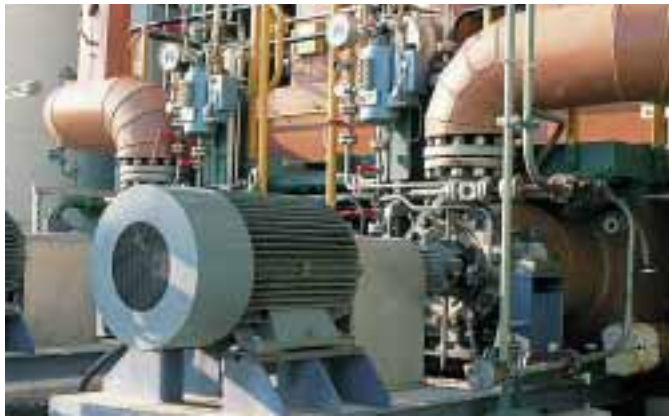
Burgmann mechanical seal type MFLWT80/S1-FD/58-E3 with thermosyphon system TS2000/M073-A1 to seal ethylene oxide (Sulzer pumps).
