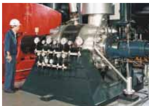
► Boiler feed pump (Weller) at the 15,000 kW Bergkamen A power station run jointly by STEAG and VEW with Burgmann type SAF2/165-E1 ( p_1 = 23.5 bar; t_1 = 163 °C; n = 5,100 min -1 ; v_g = 46 m/s)
