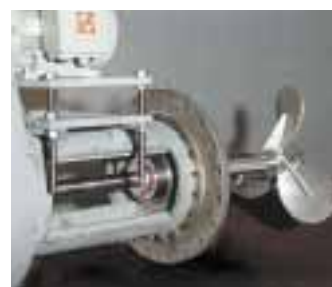
Washing suspension circulating pump (KSB-KWP) with a Burgmann type HR321/290 mechanical seal.
