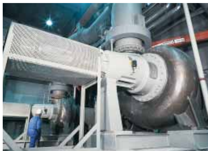
Washing suspension circulating pump (KSB-KWP) with a Burgmann type HR321/290 mechanical seal.
