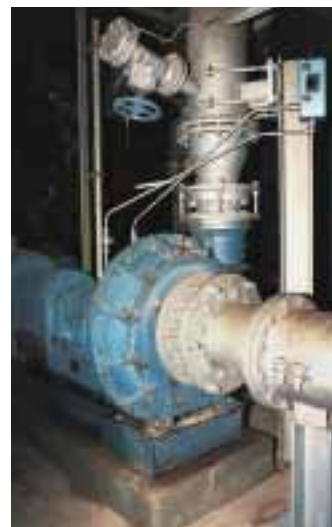
Residue evacuation pump (Habermann) with HR222 S1/140 tandem seal and QFT 2000.
