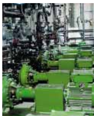
Non-clogging pumps (KSB, KWP) with Burgmann type MFL85N mechanical seals ( Q_{12}Q_1, V T_6G_1 ) in a 5-stage biological sewage works run by DEA Union-Kraftstoff AG, Wesseling, for the biochemical elimination of nitrogen in ammonium-enriched refinery waste water. The useful life of these seals in dead-end arrangement is between 3 and 4 years in the 30 pumps installed at the works. ( d_1 = 53 \dots 90 \text{ mm} ; p_1 = 2 \dots 4.5 \text{ bar} ; t = 20 \dots 40 \text{ °C} ; n = 950 \dots 1,450 \text{ min}^{-1} ).
