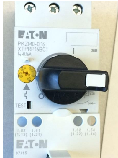
Motor Protector disconnect shown in the Open or Tripped position.
