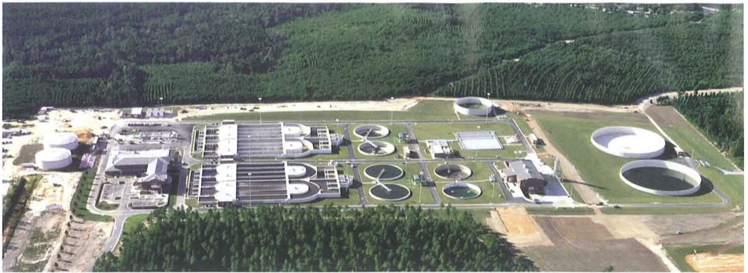
The new Central Water Reclamation Facility in Cantonment is built to be more environmentally friendly and hurricane resistant.
