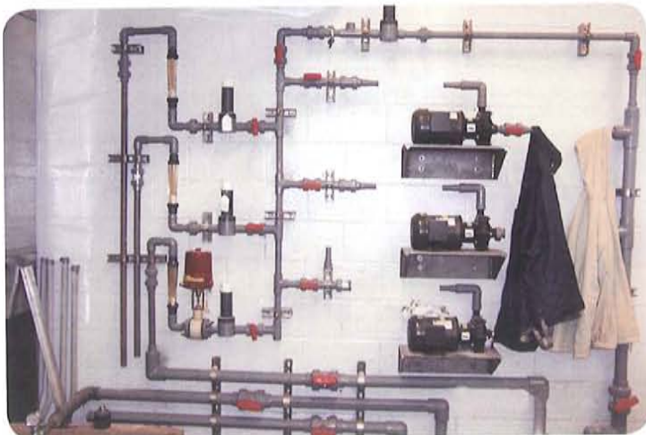
Above: Pumps inject bleach (made on site) into the disinfection basin.
