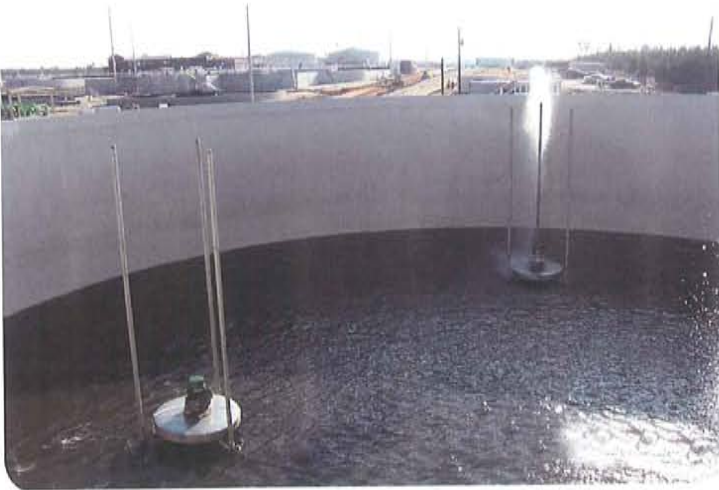
Above: During periods of high flow to the CWRW, the influent equalization or overflow basin stores excess wastewater until it can be treated.
