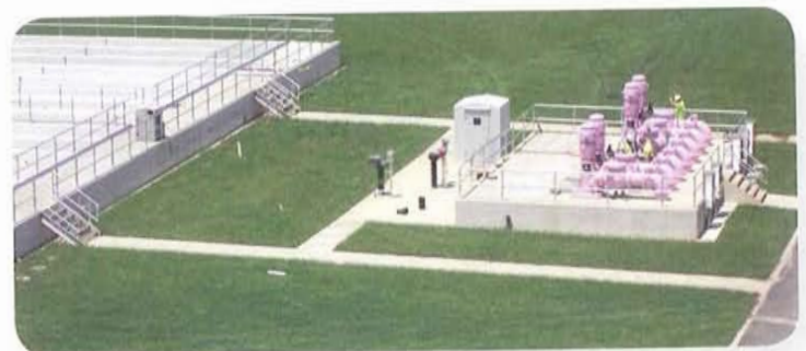
Above: Effluent pumps transfer reuse water to storage tanks on site. From there, water is sent to Gulf Power Company and International Paper.
