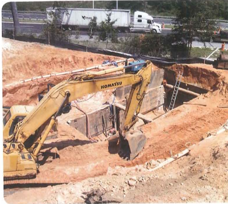
Above: Contractors prepare to auger pipe under I-10. Using the “jack and bore” technique eliminates the need to stop traffic or tear up the roads during installation.
