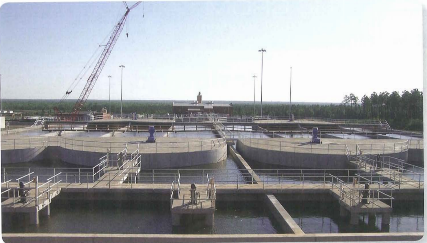
Above: Multiple stages of the biological nutrient removal process, where bacteria “eat” phosphorus and nitrogen.
