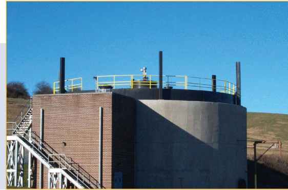
Truss Gasholder with Slide Guides
