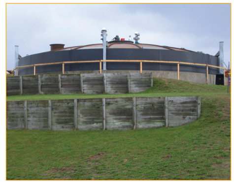
Radial Beam Gasholder with Slide Guides
