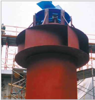
Centrifugal Impeller Pump and Draft Tube
