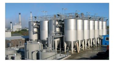
The **SuperSand™ Filter** employs a backwash rinse that is performed continually while the tank is processing water. An air lift pump located at the center of the module draws the media from the bottom of the filter up into the wash box. As the media is released into the wash box, it falls into the sand scrubber where the filtered solids are separated from the sand. From there, the filtrate carries the solids out as waste. The washed sand falls down into the media bed for continued use.
