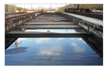
WesTech's **Oil/Water Separators** combine state-ofthe-art separation, skimming, and sludge transport technologies into a highly efficient primary oil separation device. Removing the bulk of free oils and greases from plant process water streams yields valuable hydrocarbons. Further processing downstream yields recyclable water for plant operations. We provide new as well as retrofit equipment. We offer traditional rectangular units as well as maintenance friendly, high torque, circular units.
