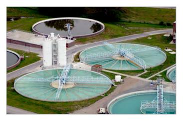
The **Solids CONTACT CLARIFIER™** is a mixture of old art and new process technology. Patent art dates back to the 1880's and contemporary solids contact clarifier units have their orginins in the 1940's and 1950's. The two most common applications of the Solids CONTACT CLARIFIER™ are cold lime softening, where the unit is used to maximize the rate of chemical precipitation, and surface water clarification, where the unit is used as an enhanced flocculation device.
