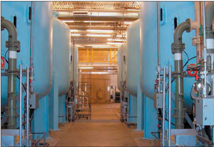
Sixteen Vertical Pressure Filters
