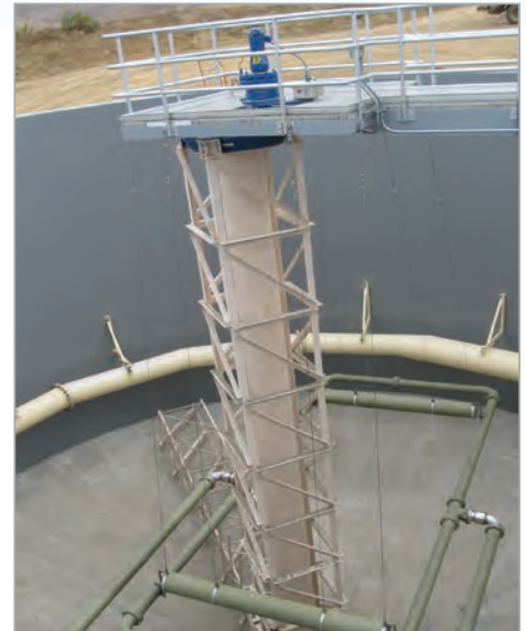
Fill and Decant Clarifier
