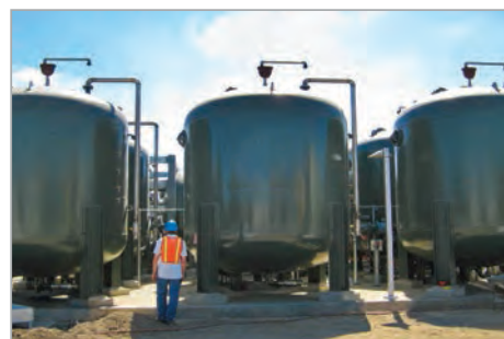
Vertical Pressure Filters at Westminster Well Site
