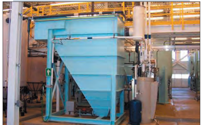
IPS\\ TM , Backwash Recovery Clarifier
