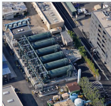
Horizontal Pressure Filters at Bundy Well Site
